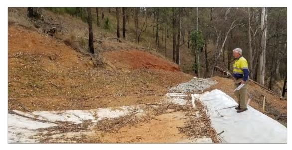
Figure 3-26 Photograph of a settling pond and lined drainage channel installed to manage rainwater run-off from drilling pads and access tracks (SRK ES Sept 2019)
